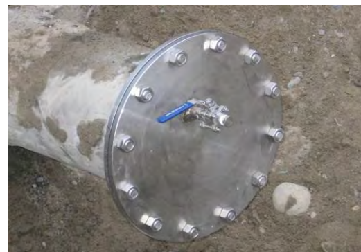
Test Slant Well Prior to Burial
