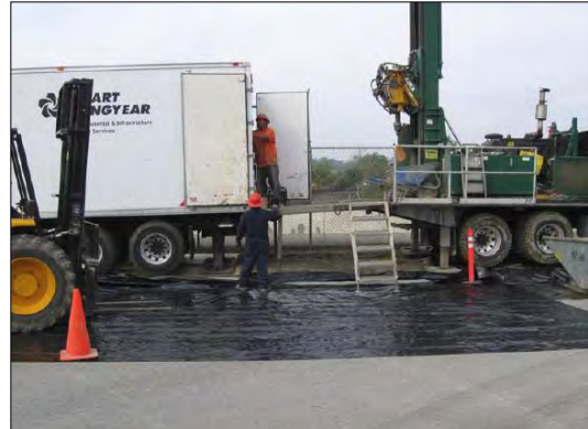
Sonic Drilling Rig with BMPs in Place
