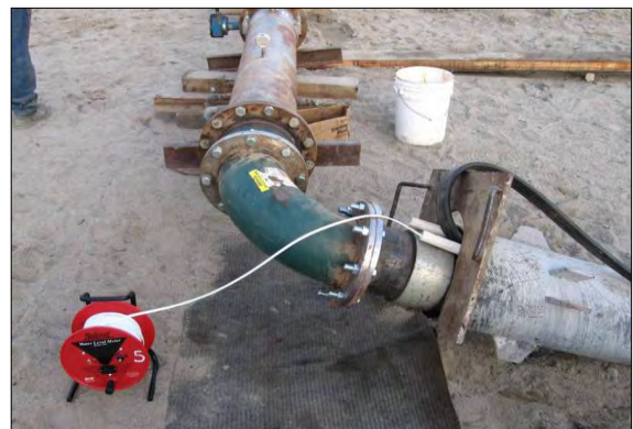
Water Level Measurement during Slant Well Testing
