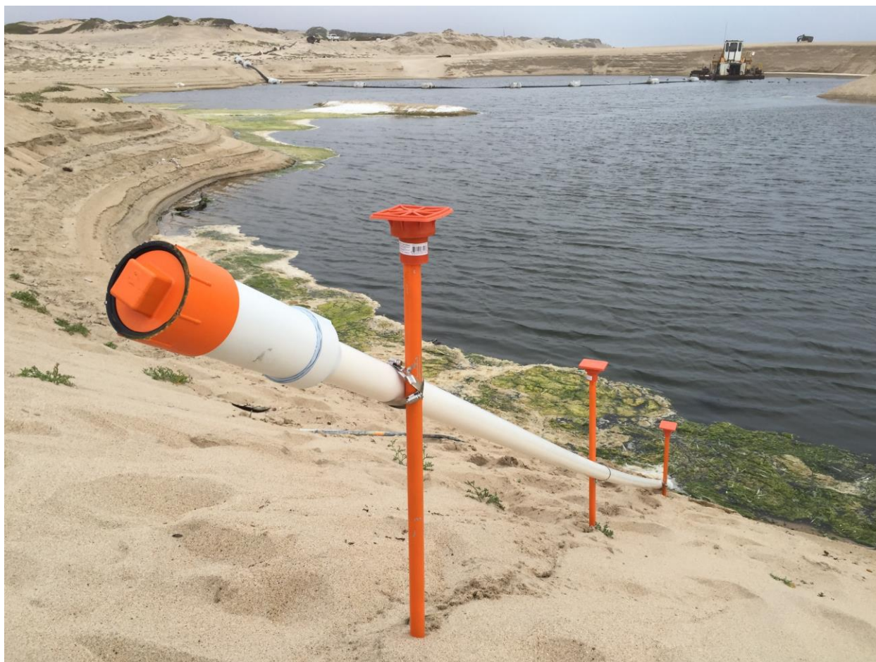
Figure 3-1. Monitoring Device – CEMEX Dredge Pond
